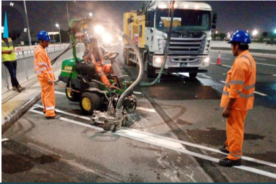
Road Marking Removal
