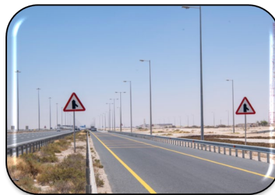
Street Light Installation
