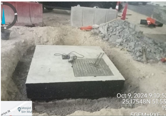
Chamber Construction
